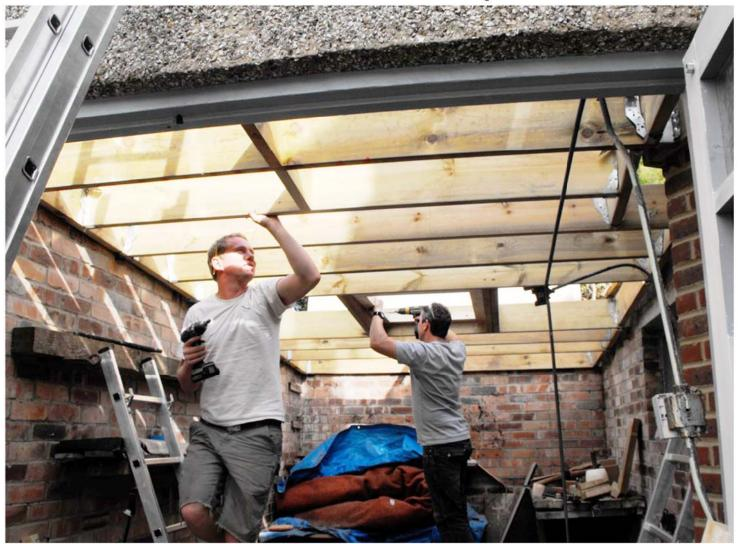
Following the pitch-line of the old roof, it was a guick process to install the new, stronger joists. Ensuring the beams and structure below are able to cope with the additional load is one of the prerequisites of green roof design. For larger structures, a structural survey should be undertaken.
