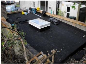
Once the ply deck was laid, the EPDM membrane is laid and dressed into the parapet walls. Here, we replaced the existing brick course with oak sleepers. On residential projects such as this it is normally possible to complete the waterproofing in a day, enabling internal works to continue undisrupted in the dry.
