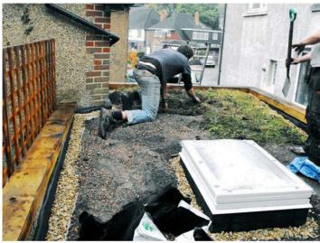
The substrate was laid in undulating fashion to better emulate the natural environment of target species. Some leftover sedum blanket was laid in one area while plugs, seeds and more developed pot plants were dotted around the roof. The perimeter and the area around the skylight were filled with creamy-coloured Cotswold chippings.
