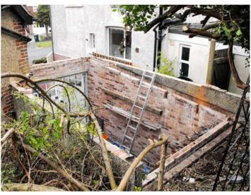
After years of neglect and encroachment by neighbouring plants the entire roof surface was condemned. Some of the joists were able to be saved for reuse as noggins, and elsewhere in the garden.
